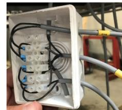
6. Serial connect the wires from the four switches according the below electrical diagram:
